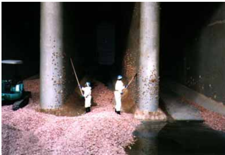
Fig. 1. Barnacles cause serious problems in electric power station.
